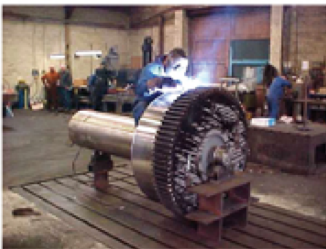
↗ Winch Core Repair.
